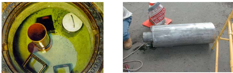
Figure 4. Dosing Siphon Top View and External Drum
