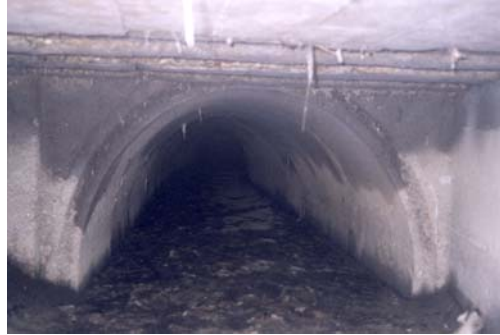
Figure 5. Wheeler Street 2.8 m Storm Drain Sewer Half Filled with Sediments
